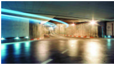
Foto: Tunnel connection to the Interchange
